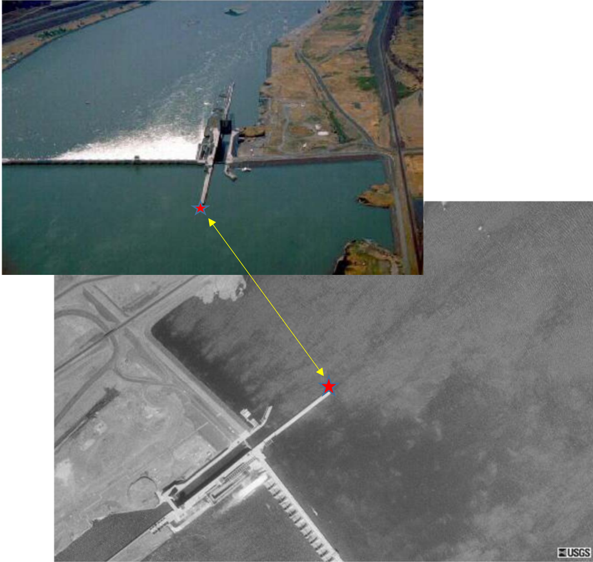
FIGURE 4. PHOTOGRAPH OF THE APPROXIMATE LOCATION OF THE JOHN DAY FOREBAY FMS GAUGE.
