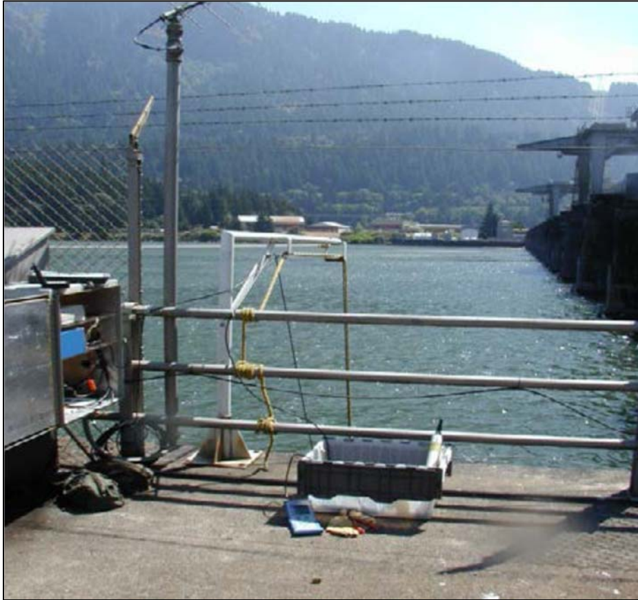
FIGURE 1. PHOTOGRAPH OF THE BONNEVILLE FOREBAY FMS GAUGE.
